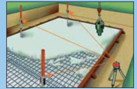
Leveling work on ceiling and floor panels
